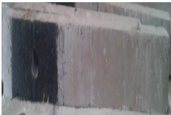
Fig. 2: CFRP wrapping around the opening
