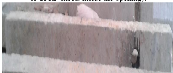
Fig. 3: CFRP wrapping inside the opening
