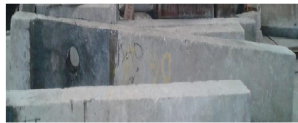
Fig.4: CFRP wrapping around and inside the opening
